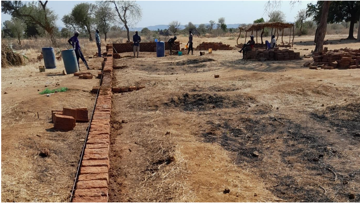
The foundation has been established
